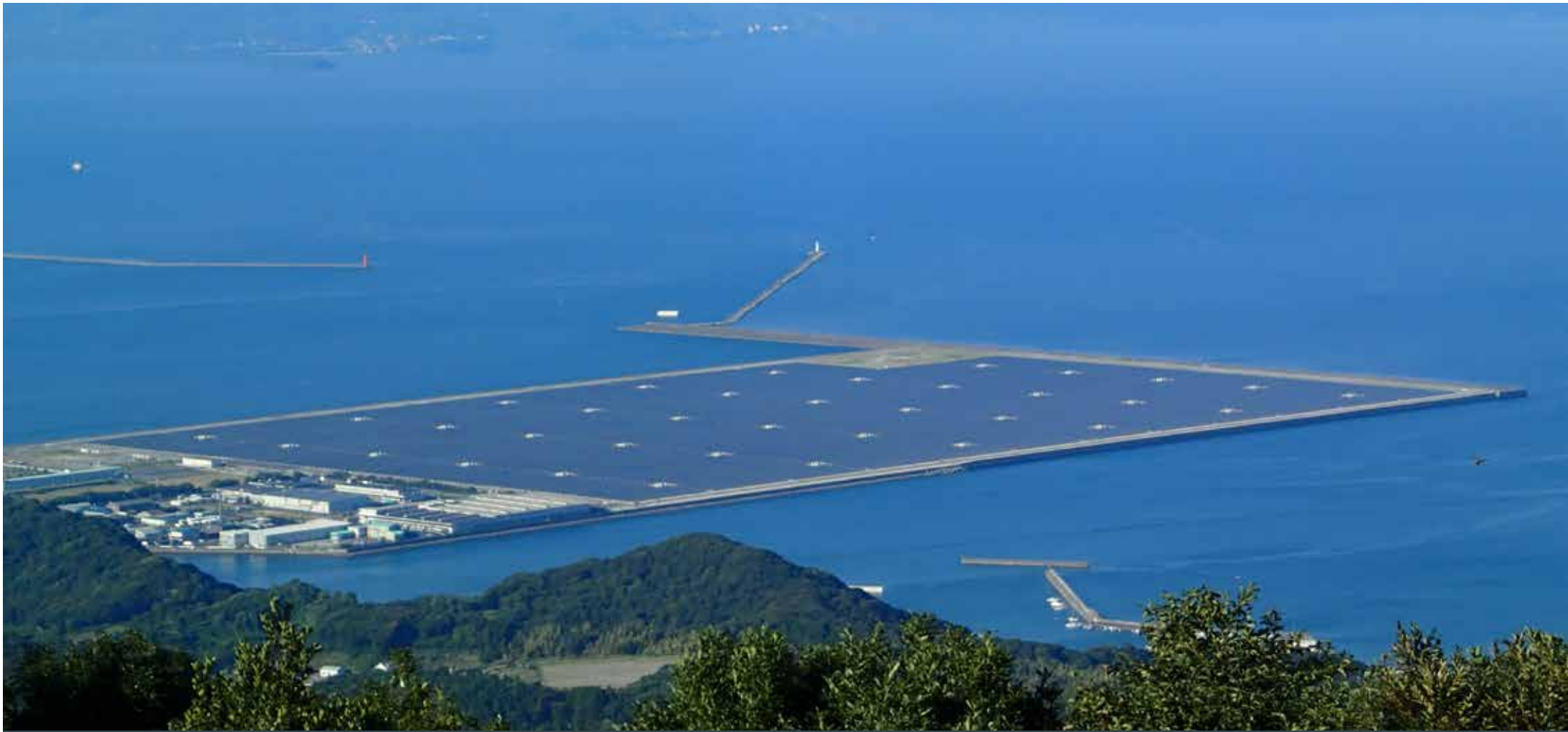
KAGOSHIMA NANATSUJIMA MEGA-SOLAR POWER PLANT
