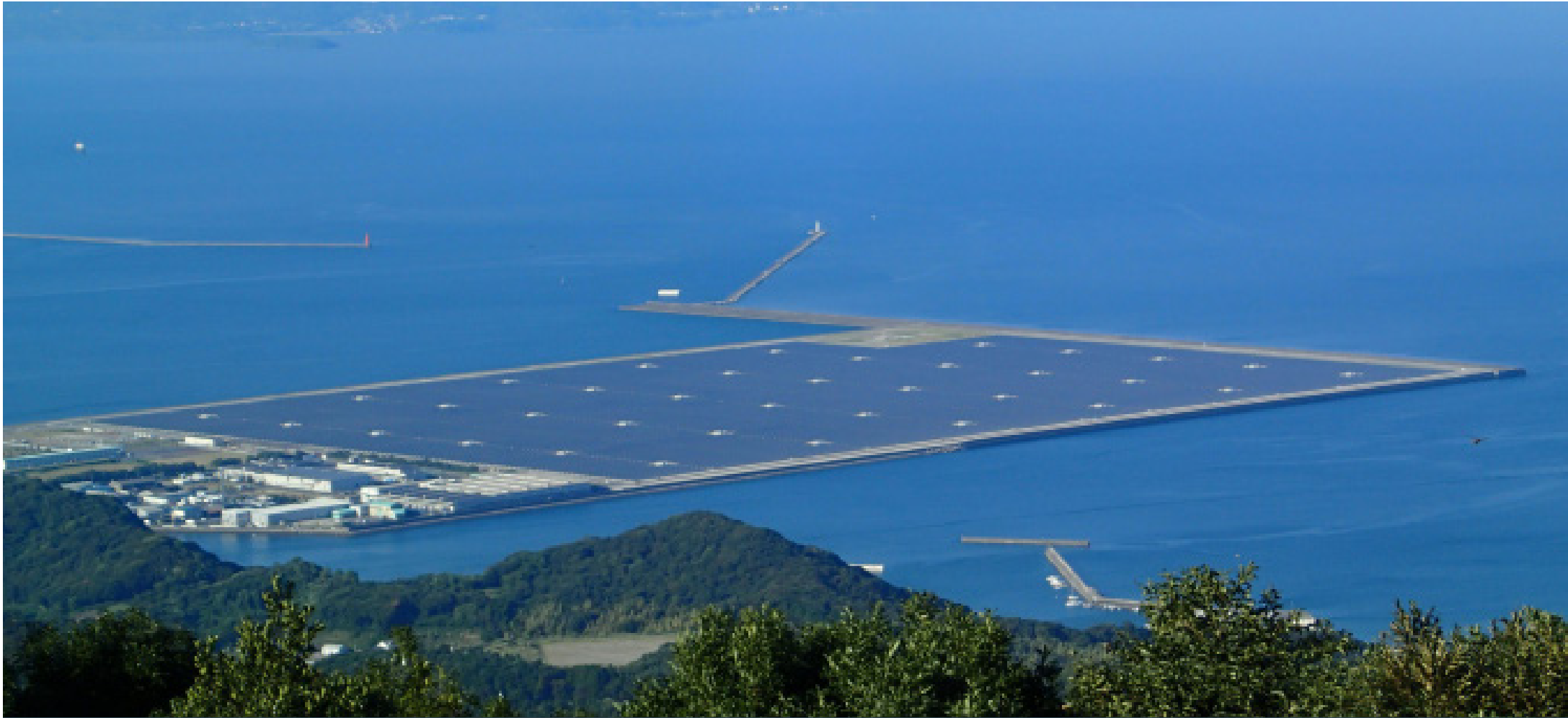
KAGOSHIMA NANATSUJIMA MEGA-SOLAR POWER PLANT
