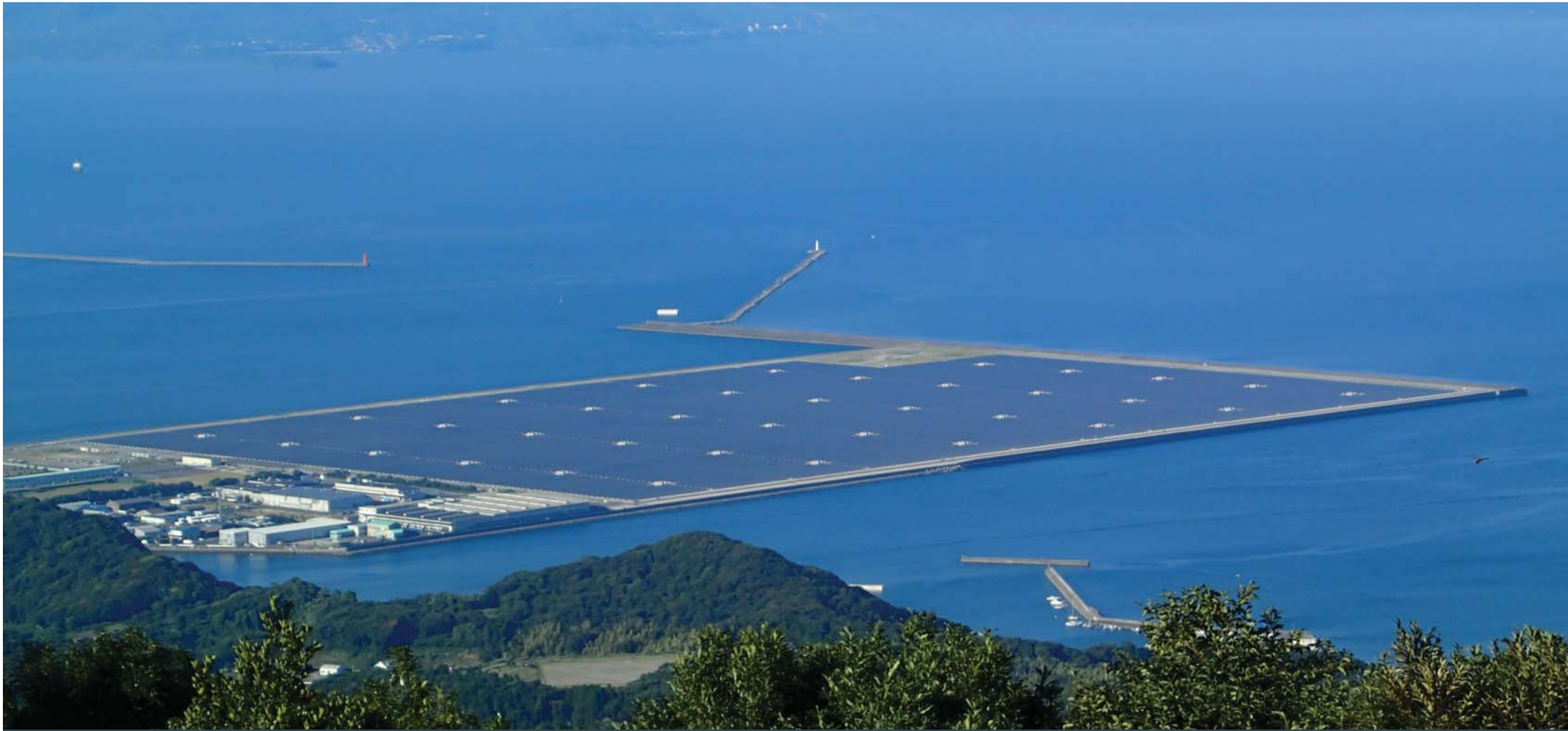
KAGOSHIMA NANATSUJIMA MEGA-SOLAR POWER PLANT
