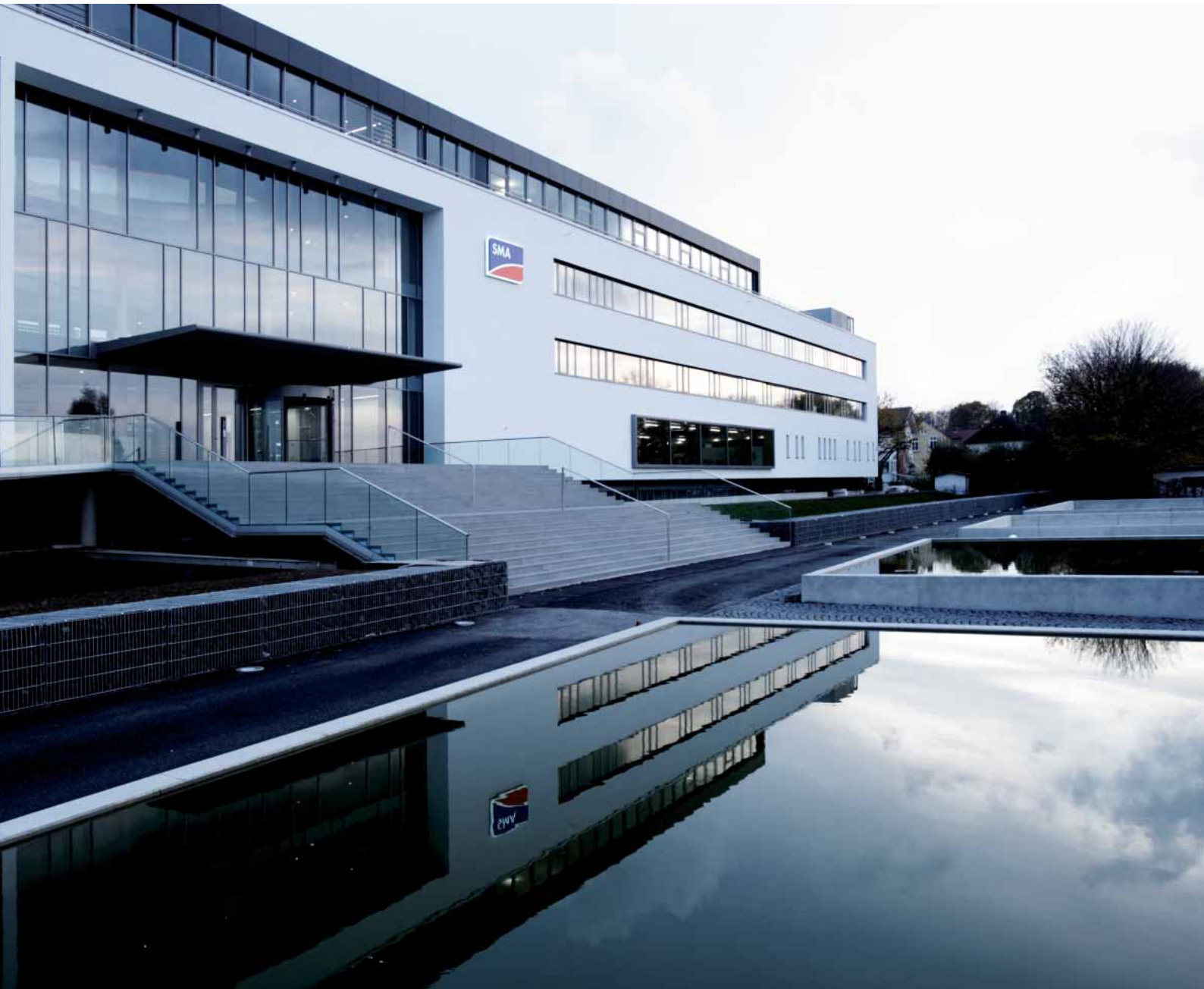
New main entrance of Sonnenallee 1 in Niestetal
